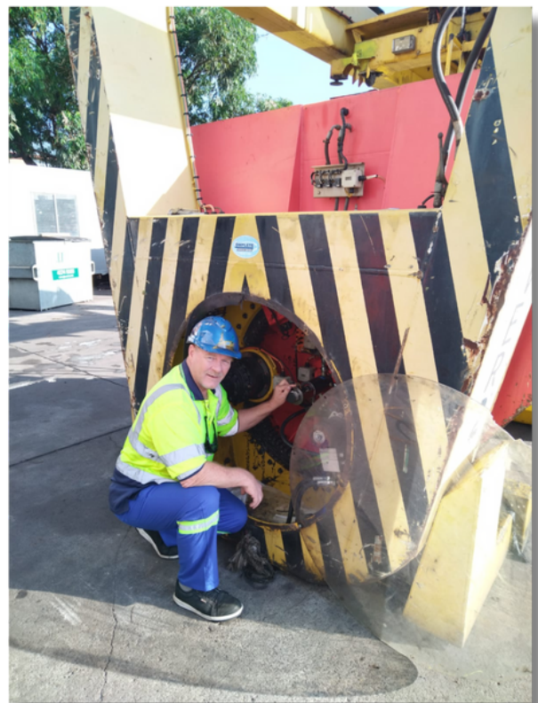
RAM Revolver refurbishment
