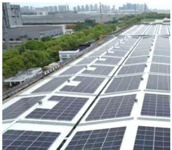
Pictured: Installation completed at RAM's manufacturing facility in Changshu, China
